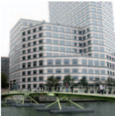
A typical 1980s to present building
