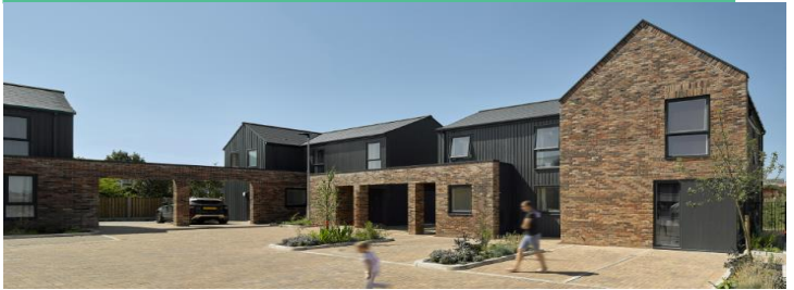
Each house type is bespoke around a communal courtyard, encouraging interaction between residents
